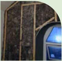
2. Glass Mineral Wool Insulation material is added to the wall inside a newly built XPS bonded to OSB frame for structure.
