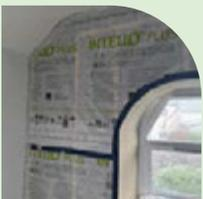
3. A vapour control layer is used to cover the insulation which prevents moisture build up.
