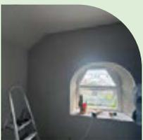
4. Plasterboard is used to cover the insulation material and serves as the final internal finishing layer, covering the insulation system and providing a smooth surface.
